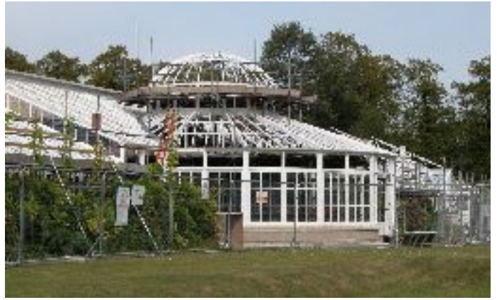
Conservatory renovation nearing completion
