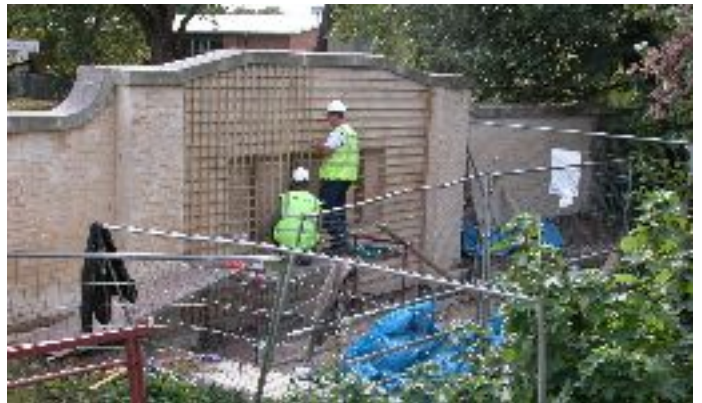
Restoring the wall and bridge behind the Southern Pool
