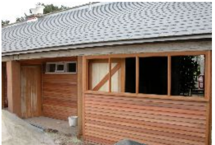
New Estate Office and facilities behind the Conservatory
