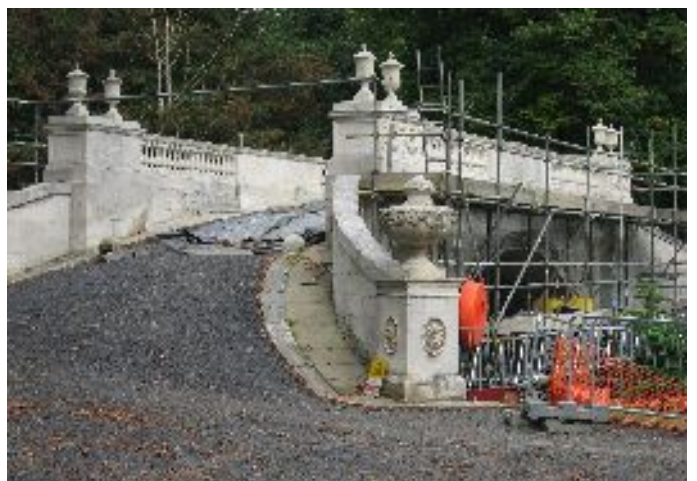
Repairs and access improvements for the Classic Bridge
