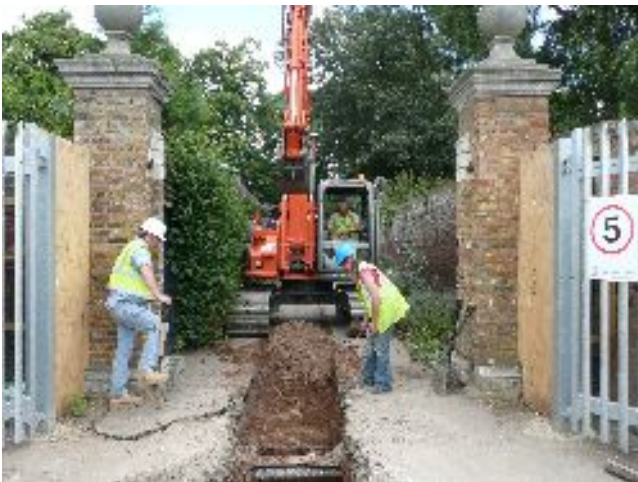
Trenching for service pipes and cables in the yard
