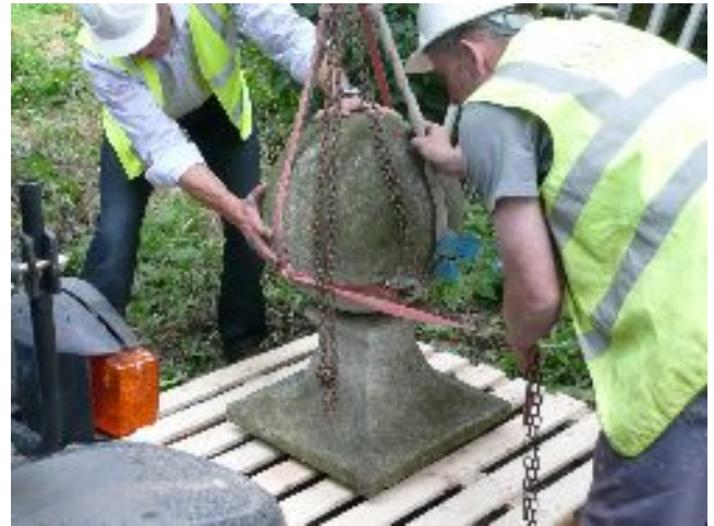
Careful handling of the gate-post masonry
