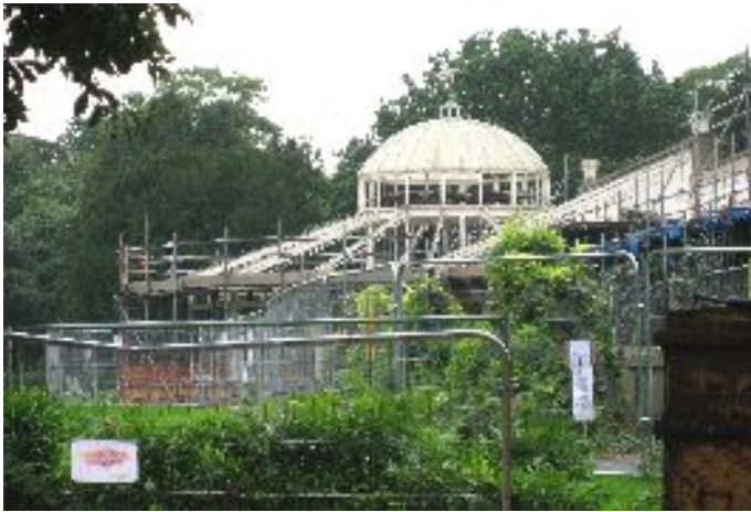
Dismantling the Camellia House
